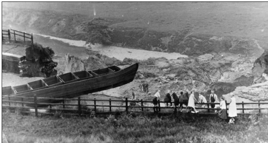
Figure 9 – The 1936 Manchester, Bolton and Bury Canal Breach
